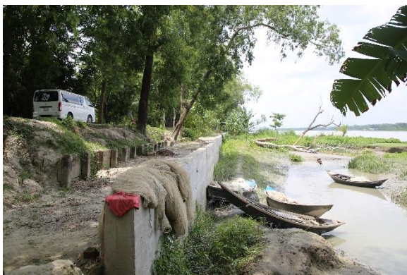
Figure 2.11: Flood Protection Work by LGED
