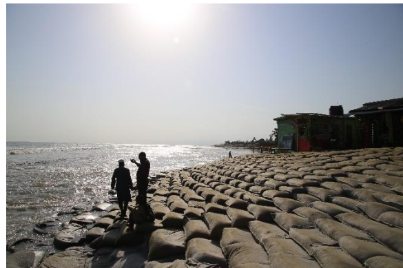
Figure 2.10: Beach Protection Work at Kuakata SEA Beach By BWDB
